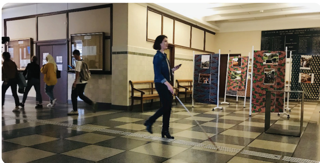
Photo 3. Floor with tactile paths near the entrance/exit
